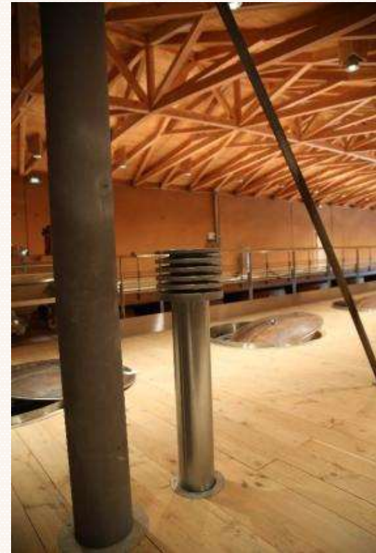
Indoor air diffuser
